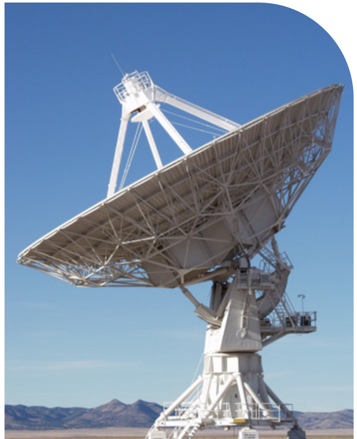
FIG 1 | A Traditional Parabolic Antenna with Mechanical Positioning to Track or Target a Satellite in Orbit
